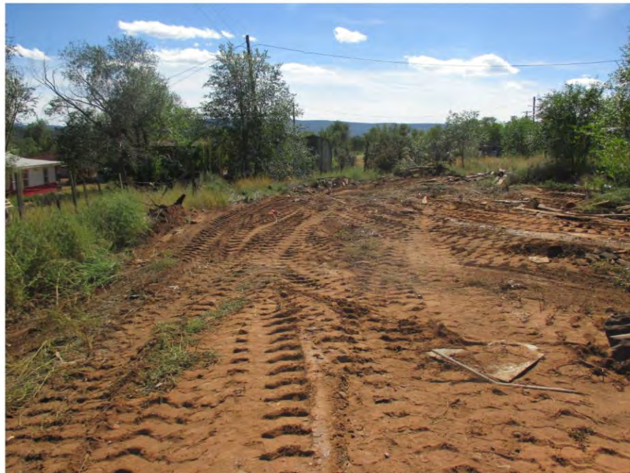
Theda Quay, Whiteriver behind WR Assembly of God Church – structure unsafe to public.
